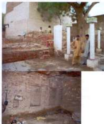
View of Ceramics and Bricks crumbling due to high humidity
