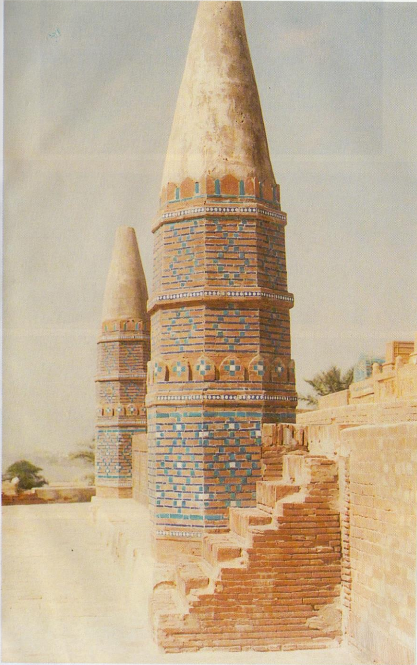
Ornamental tower, lightly studded with glazed brick pieces, has decorative bands, the Kungra (battlements) band creat quite an impact. Sufa-e-safa , Rohri.
