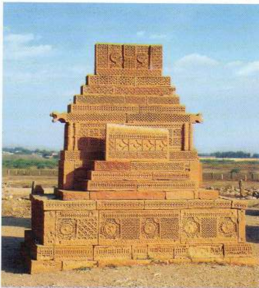
Picture U: The platform added height to the grave, Chukhandi graveyard.
